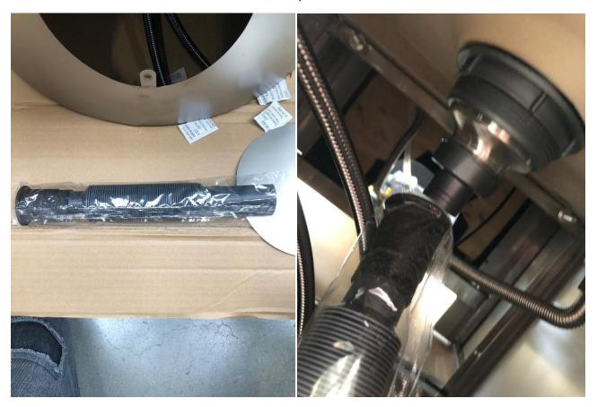
4. Connect the tube to the steam generating device as shown in the illustration.
